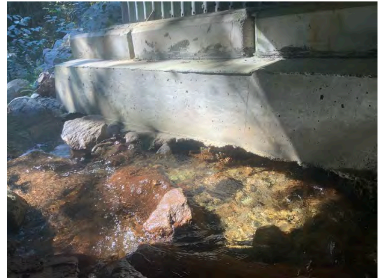
Right Bank Abutment when facing downstream
